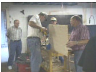
In this picture, we're drilling the pocket holes in the bottom panel of the cabinet. The new model K-3 Kreg Jig makes this
